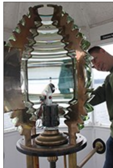
Chad Kaiser cleaning the active 4th order Fresnel lens in the lighthouse tower.
