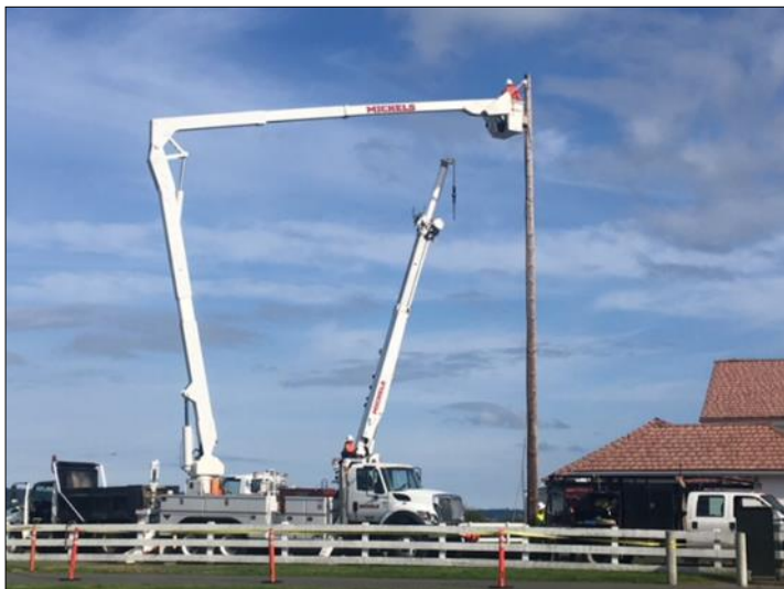
USCG Vendors Replacing the Antenna and Wooden Pole.
