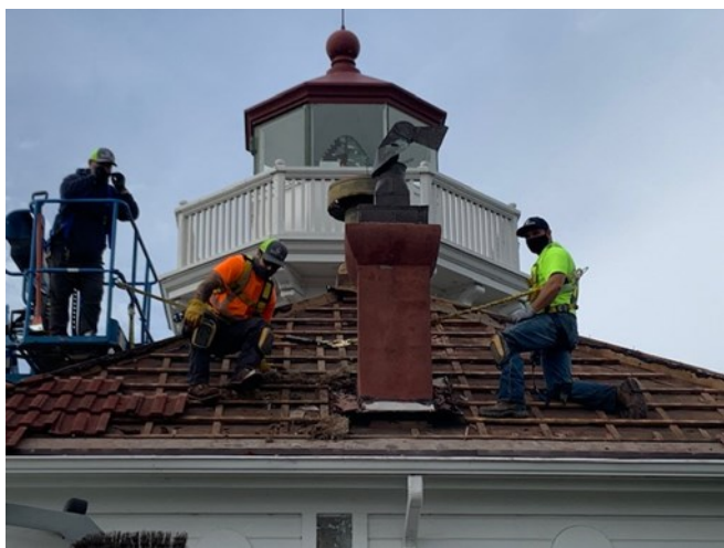
Public Works personnel removing old concrete tiles.
